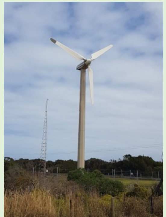
WT with one tip spoiler deployed, monitoring tower behind with 10m and 22m anemometers.
