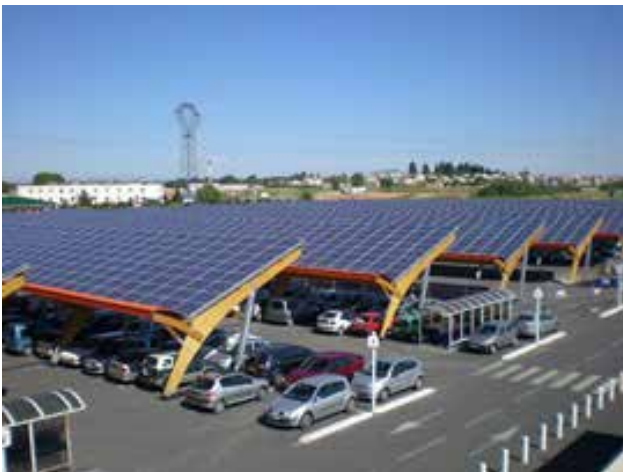
Figure 3: Solar modules integrated into the awnings of a shopping centre in St Aunès, France. The 1.15 MWp system comprises 12 shading structures, each of which is 85 m in length, and shade 816 car spaces while reducing the air conditioning bill of the shopping centre. (Source: Sunvie.)
