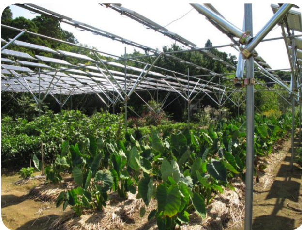
Figure 2: Solar array and crop at the 34.4kW Kazusaturumai Solar Sharing Project
