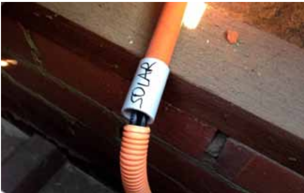
Figure 5: This is a common problem found with conduit work. Conduit connections need to be glued and firmly fixed in place so that they will not come apart.
