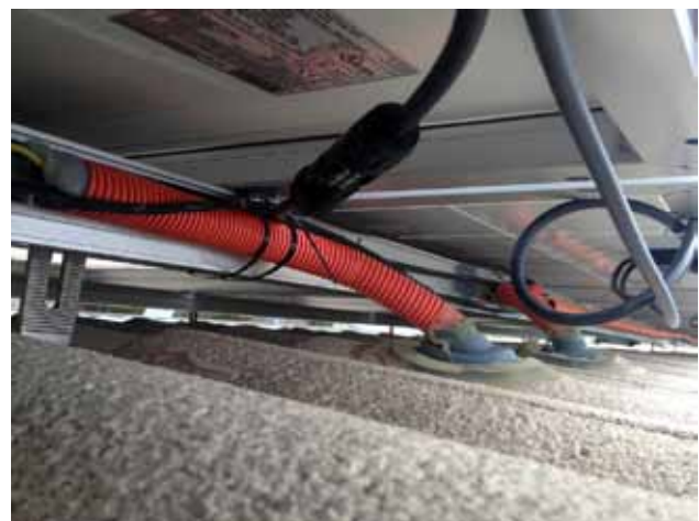
Figure 4: Non-UV resistant conduit under PV modules is exposed to reflected UV, and the conduit may degrade over time.
