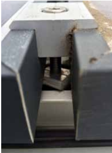
Figure 8: An incorrectly installed keystone. It is vital the clamps are properly aligned when they are installed or they will not adequately secure the modules.
