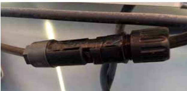
Figure 6: These connectors mated together are from different manufacturers. This may lead to a dangerous hot joint.
