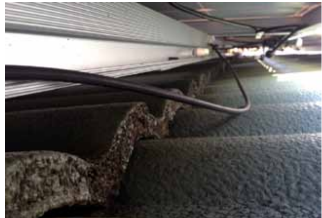
Figure 2: Cables resting of the roof can rub over time and wear away the cable insulation.
