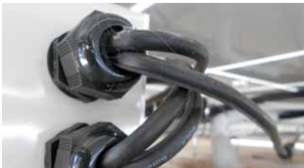
Figure 3: Water is known to run along cabling, so it is important that glands fit tightly around each cable. If a single cable gland is used for multiply cables, like in this picture, water might be able to leak through.
